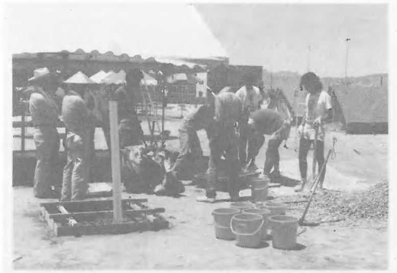
Fig. 7. The construction of the concrete base for the telescope.
